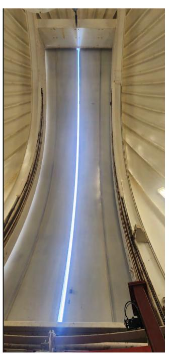
This image shows that the doors are not closing parallel, which supports the theory that the clamping mechanisms at the top are loose.
